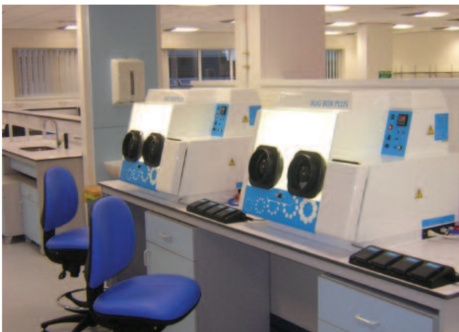
Bug Box Plus workstations installed in the new Pennine microbiology laboratory.
